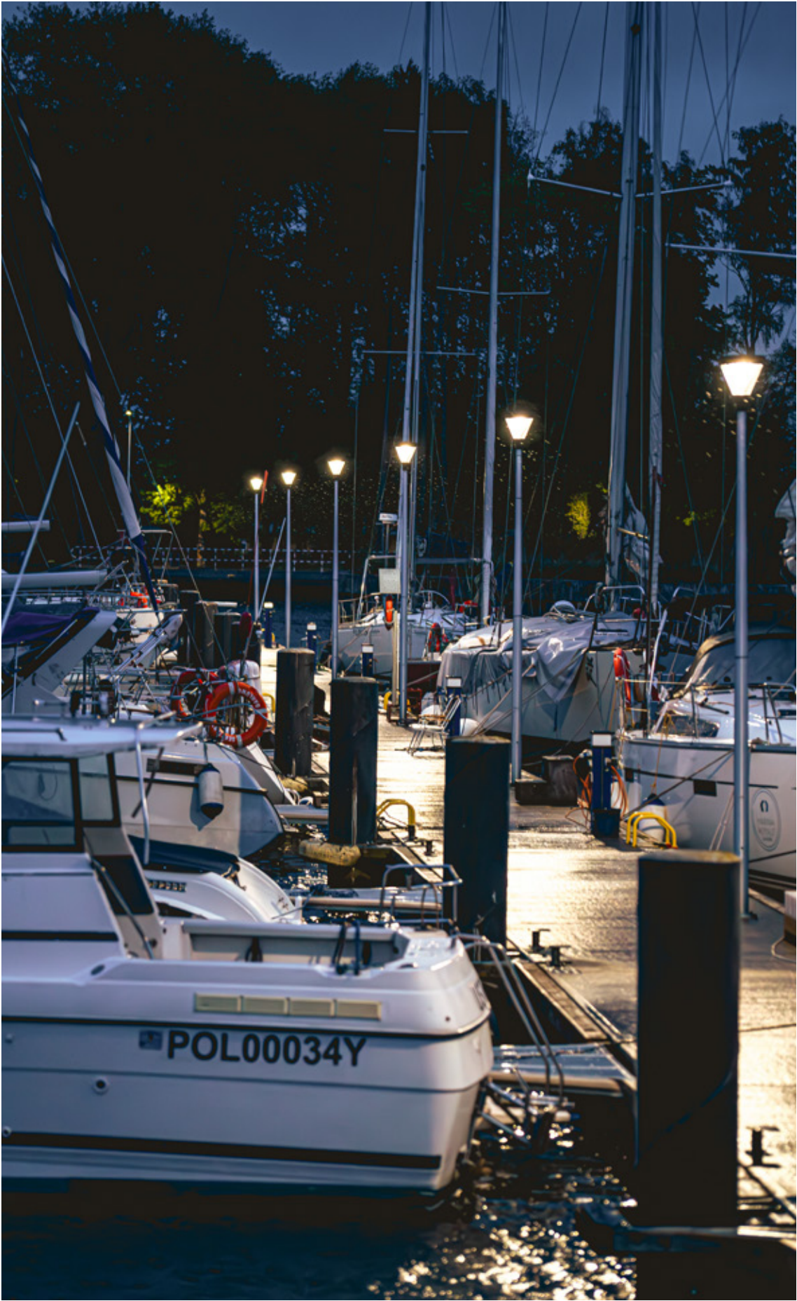
Skver LED lighting in the port
