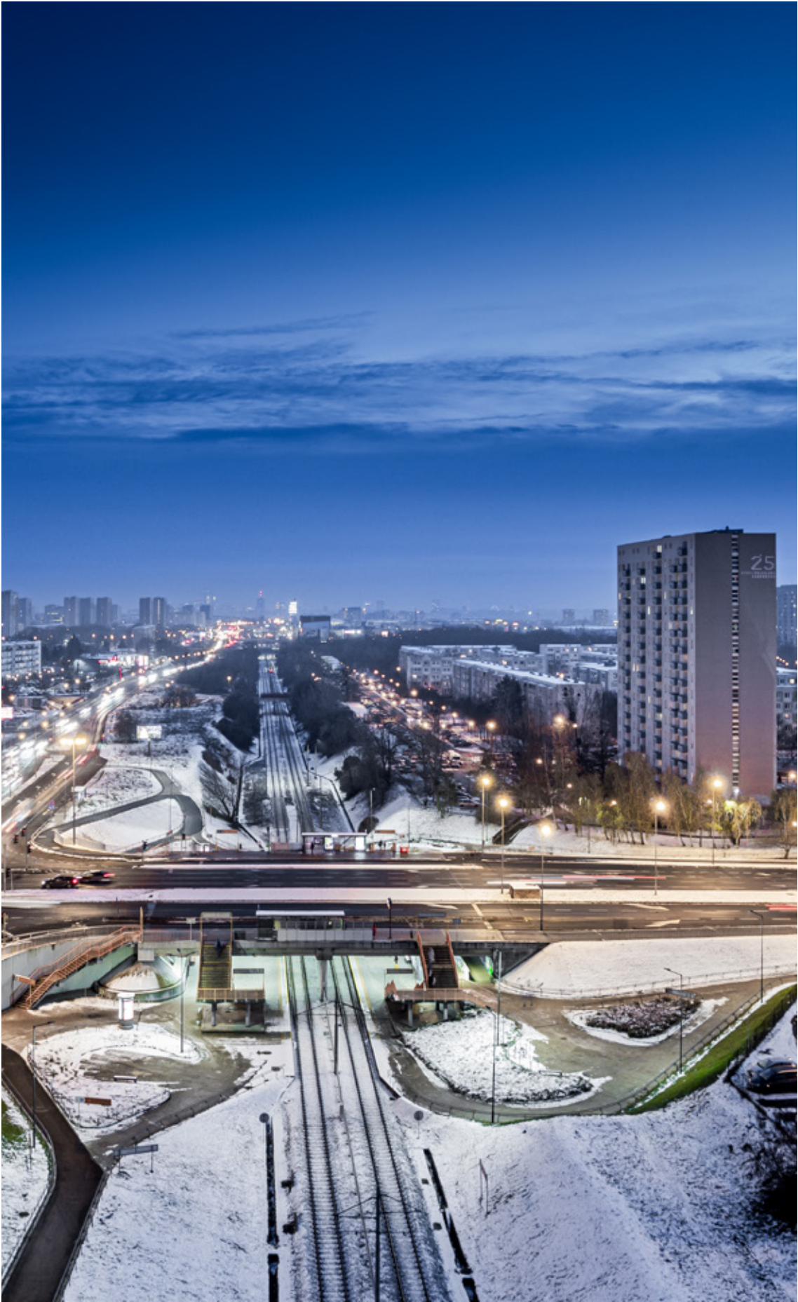
Poznań road lighting
