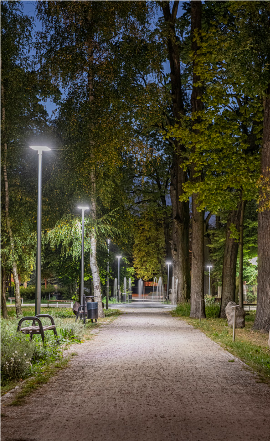
Mitra LED luminaires in the park
