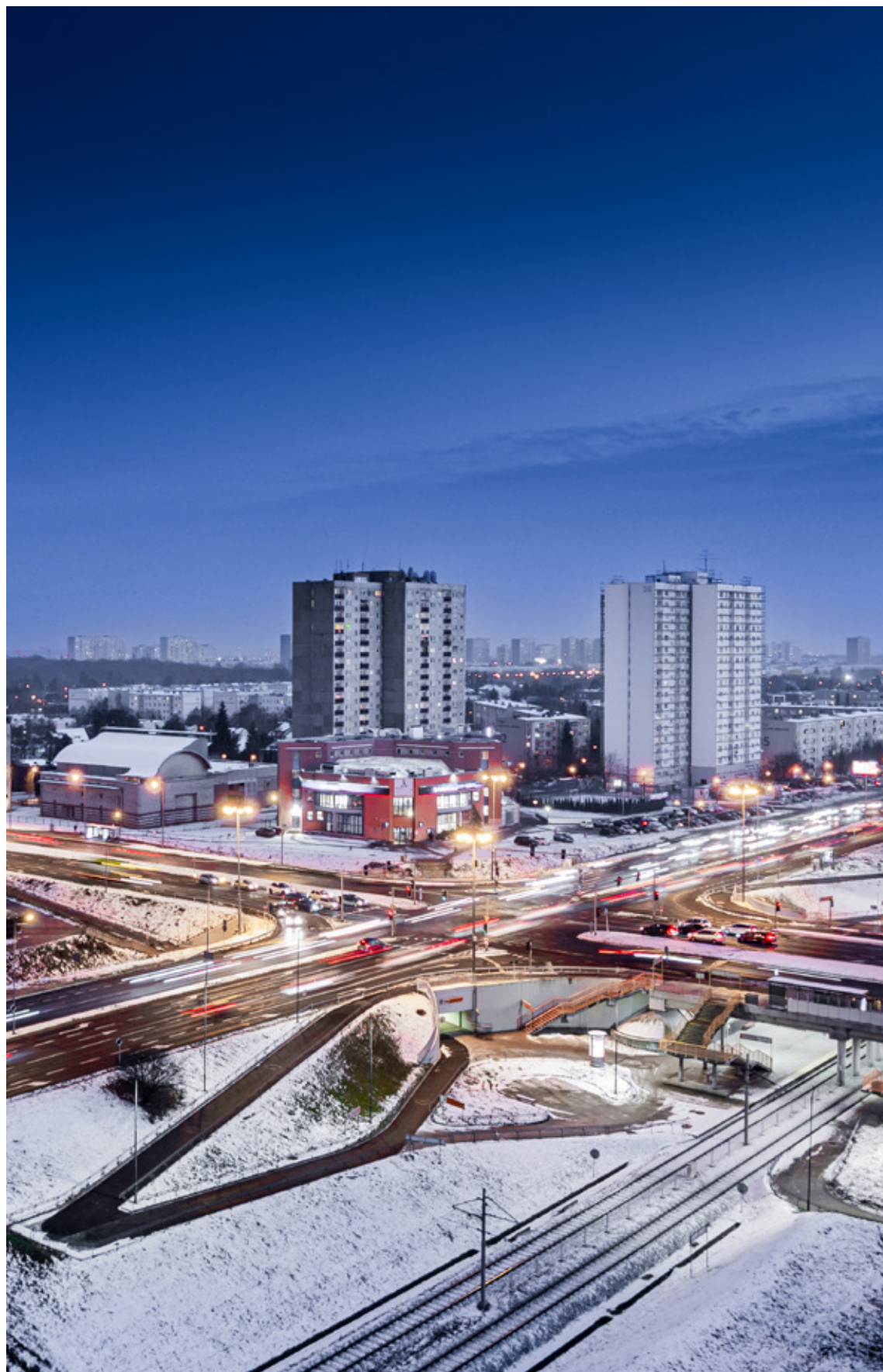
Tiara 2 LED luminaires, MPK Poznań depot
