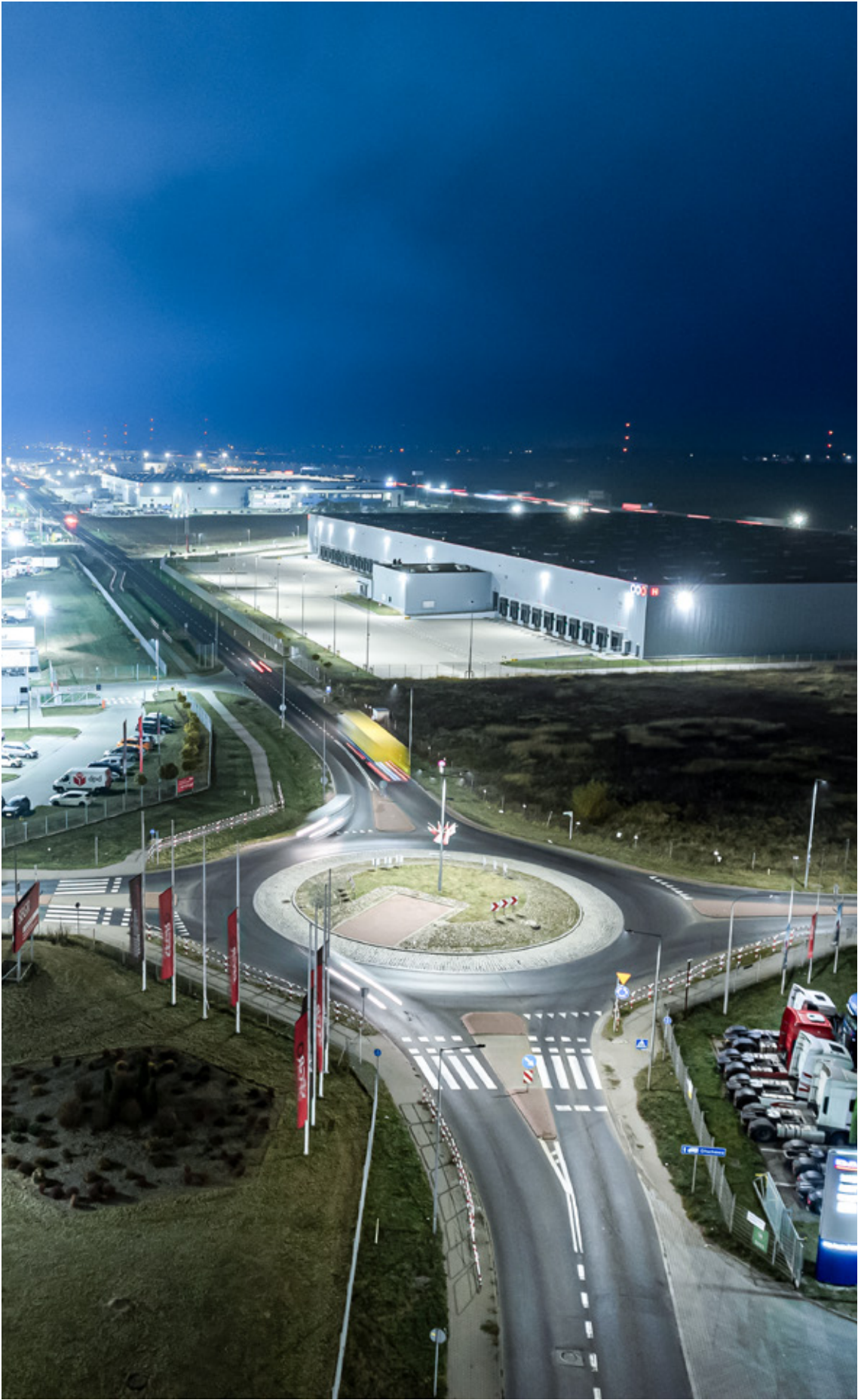
The use of Astra LED Alu luminaires
