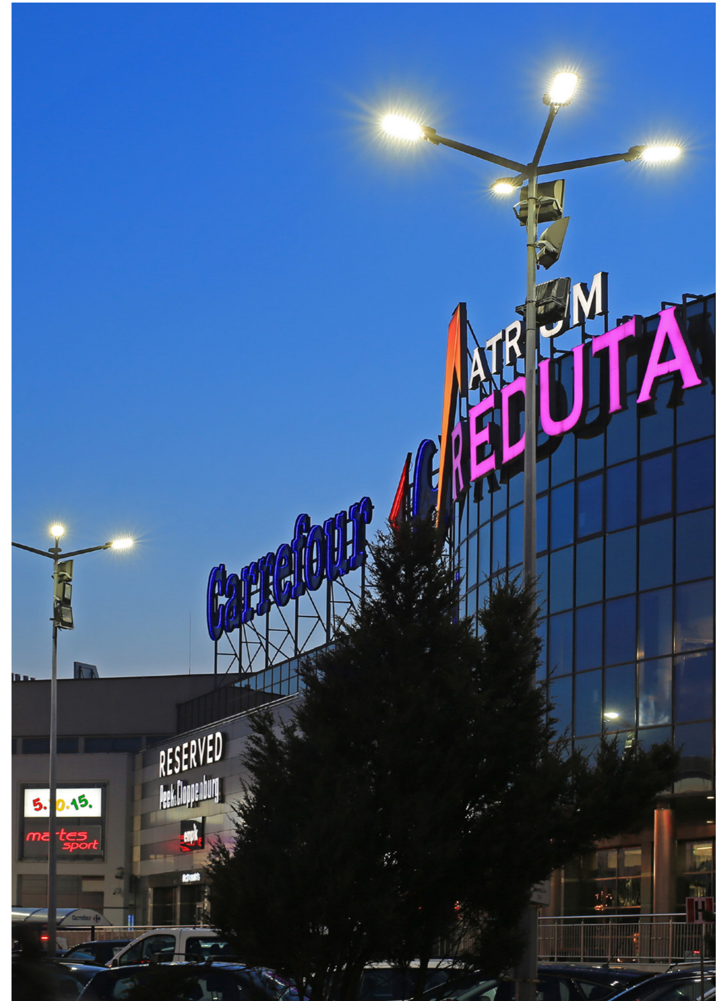
The use of the Astra LED luminaire in the parking lot in front of the "Reduta" Shopping Mall in Warsaw
